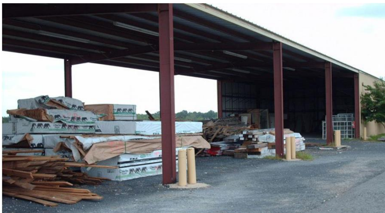
Figure 3. TIPS Warehouse, Huntsville, TX
